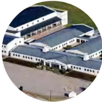
Curro Langebaan Independent School in the Western Cape
